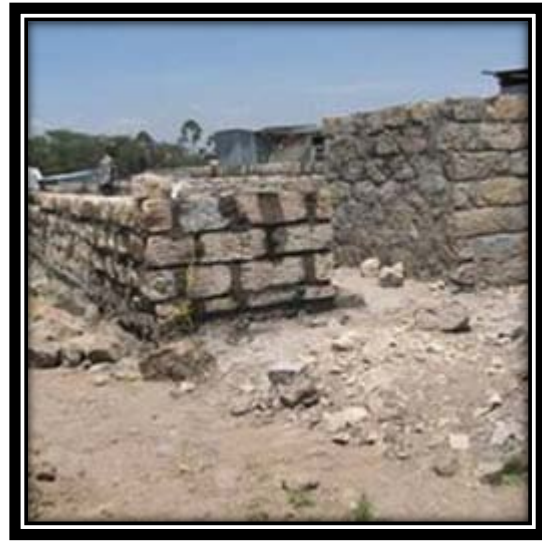
Construction of a new house in KCC, Nairobi
